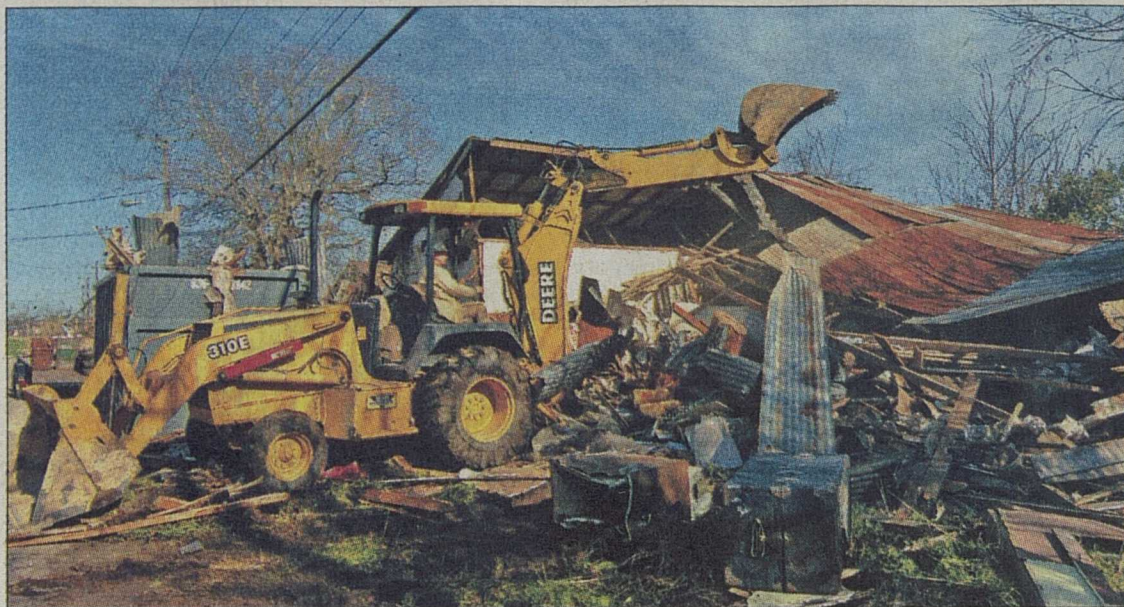
The city took another step toward getting Eagle Lake cleaned-up last week when they tore down a dilapidated home on C Street. The city says more demolitions of dilapidated or dangerous structures will come when funds are available. The city currently has one more property ready for demo on Clark Street.
